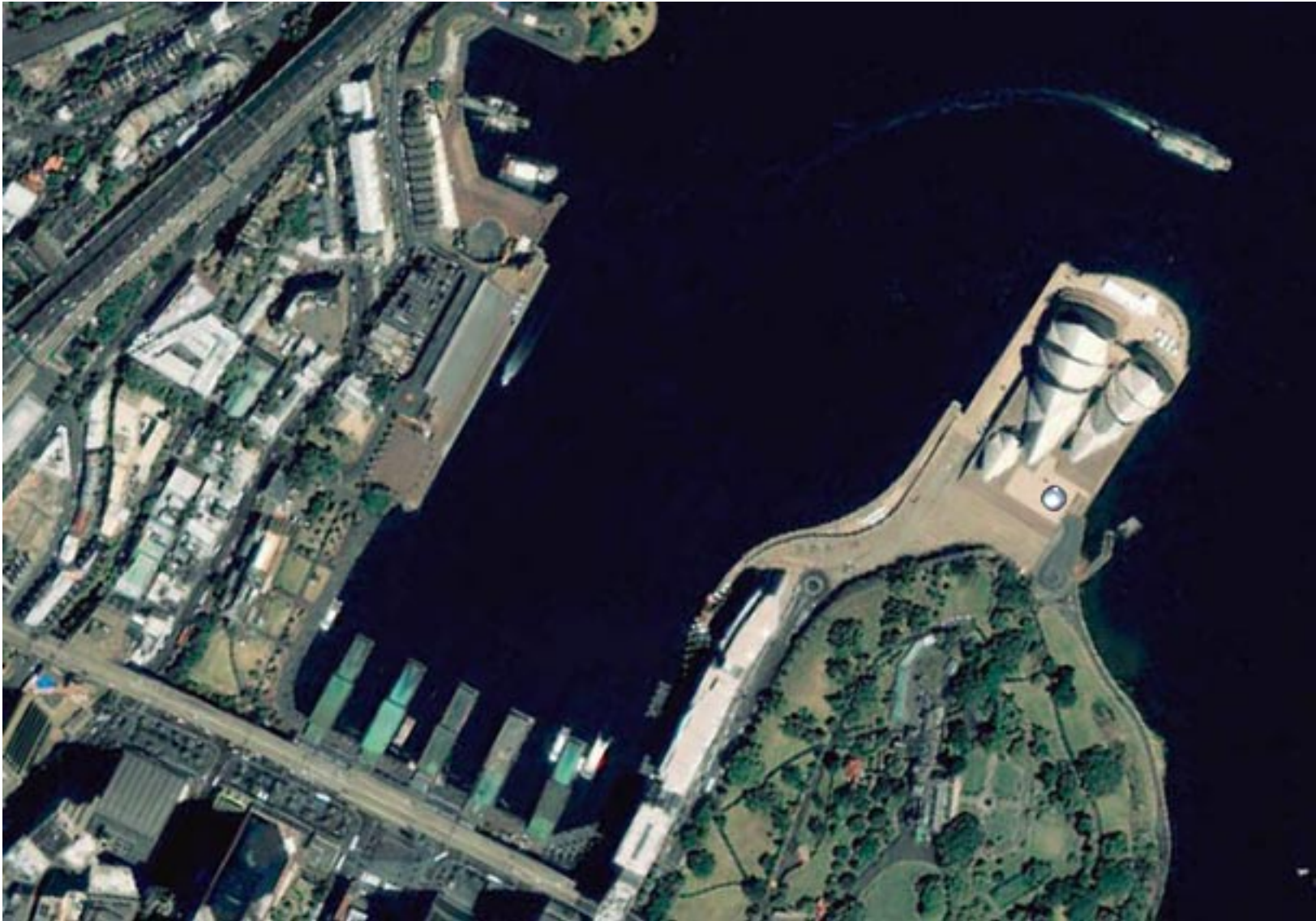
The Sydney Opera House - Australia
